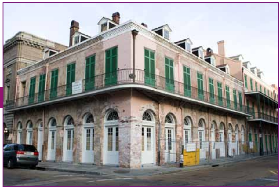
A recent view of the building under construction, December 16, 2009
